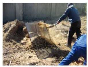
Fig. 5.10 Pebbles and stones being removed from sand by sieving
